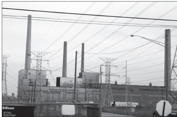
A coal-fired power plant in the US. Industrialised countries' coal use is projected by the International Energy Agency to drop by a third in the next 20 years.
