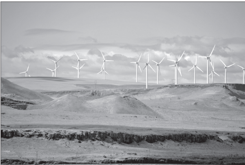
A wind farm in the United States. Wind farms can be installed much faster and typically at lower cost than new nuclear plants.
