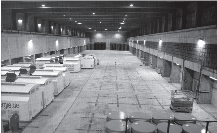
A temporary nuclear waste storage facility in Gorleben, Germany. The proper disposal of nuclear waste is one of the many problems posed by atomic energy.
